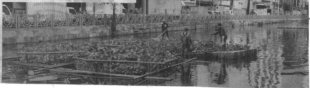
THE Pasig River Rehabilitation Commission river warriors remove heavy metals and other solid waste suspended in the water hyacinth floating wetland, a phytoremediation system to improve the water quality of Estero de Binondo. PRRC PHOTO
