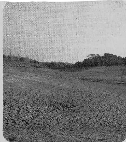
■ Dessication cracks at the sides of the reservoir.
