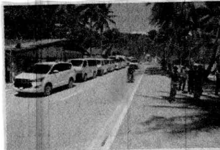
A SEGMENT of the rehabilitated Boracay circumferential road as of March 18. DPWH
